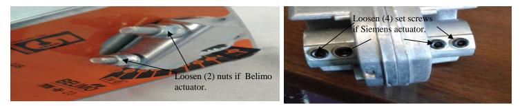
usually located on the outside of the air duct, but could be internally mounted inside the duct. The shaft clamp is secured with set screws (Siemens) or U-clamp (Belimo) with nuts, depending on the type of motor used.
