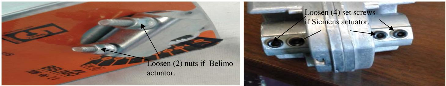
usually located on the outside of the air duct, but could be internally mounted inside the duct. The shaft clamp is secured with set screws (Siemens) or U-clamp (Belimo) with nuts, depending on the type of motor used.
